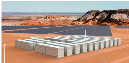
8 MWh VRFB to support a 6 MW solar array Hawker, South Australia
