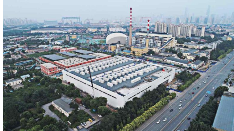
Dalian flow battery Station 800MWh - increased grid stability and backup power
